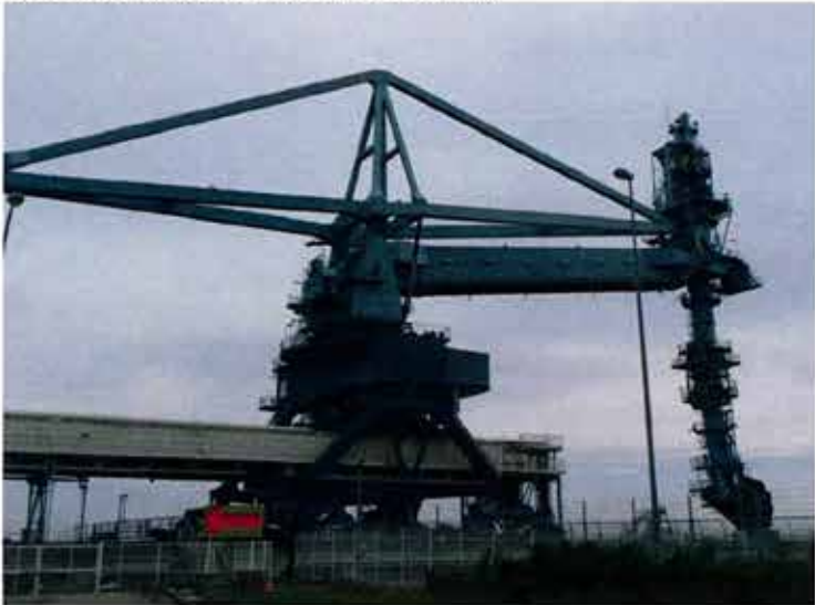
Unloader (Thermal power station)
